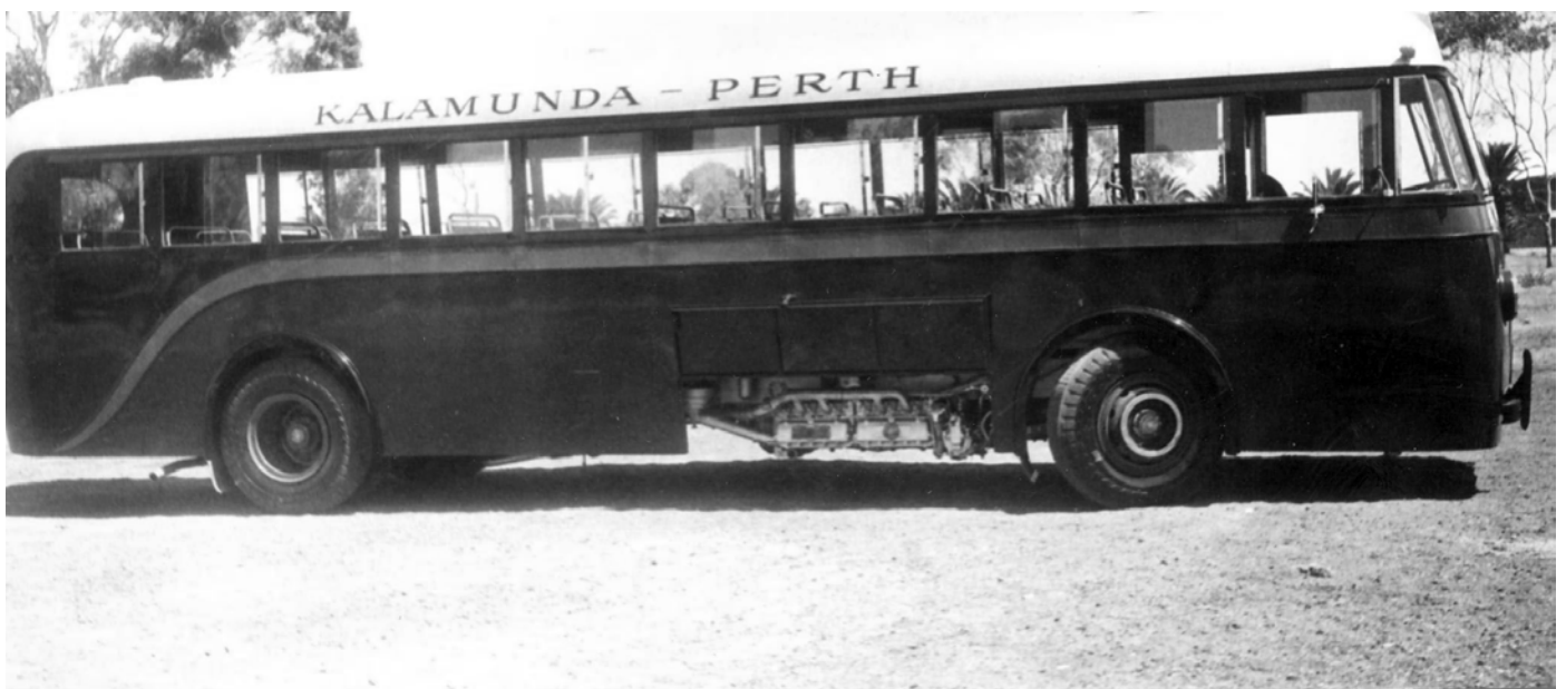
Figure 2. Mid-underfloor engine 1952
